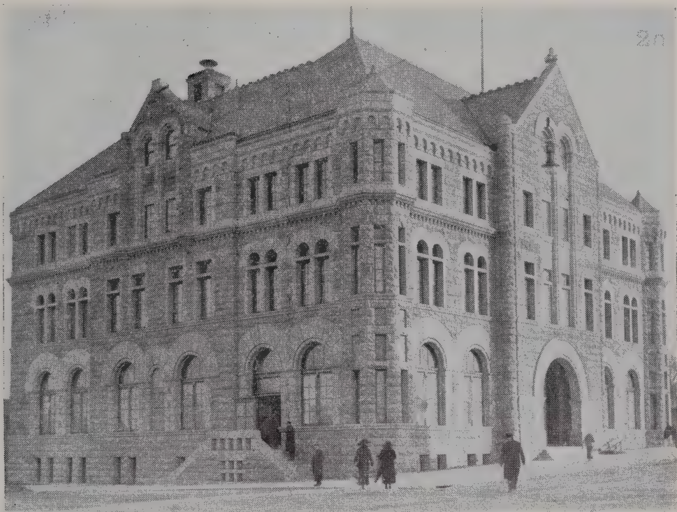
Postoffice Building, third story added
