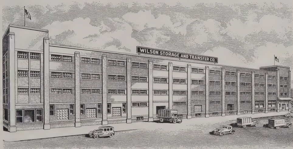
Wilson Transfer and Terminal Building.
