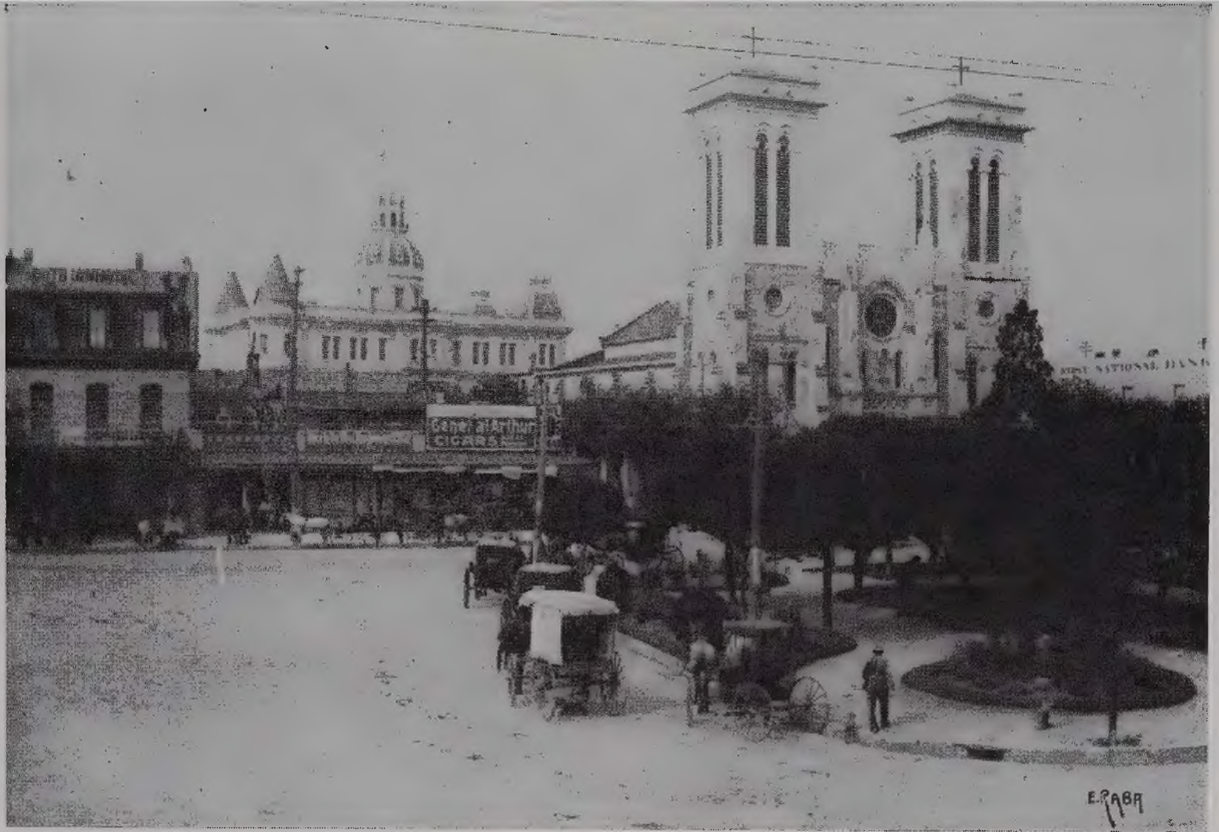
San Fernando Cathedral and Main Plaza looking west in 1902. The city hall, built in 1888-1892, is in the background, a Renaissance-style building. The Southern Hotel is at the left. The old San Pedro ditch ran in front of the Cathedral, and hotel guests and town boys used to fish off the hotel porch. Hacks, fancy importations from Europe, costing as much as $1,600, made their stands on the plazas, for rides about the city and to the missions. © E. Raba.
