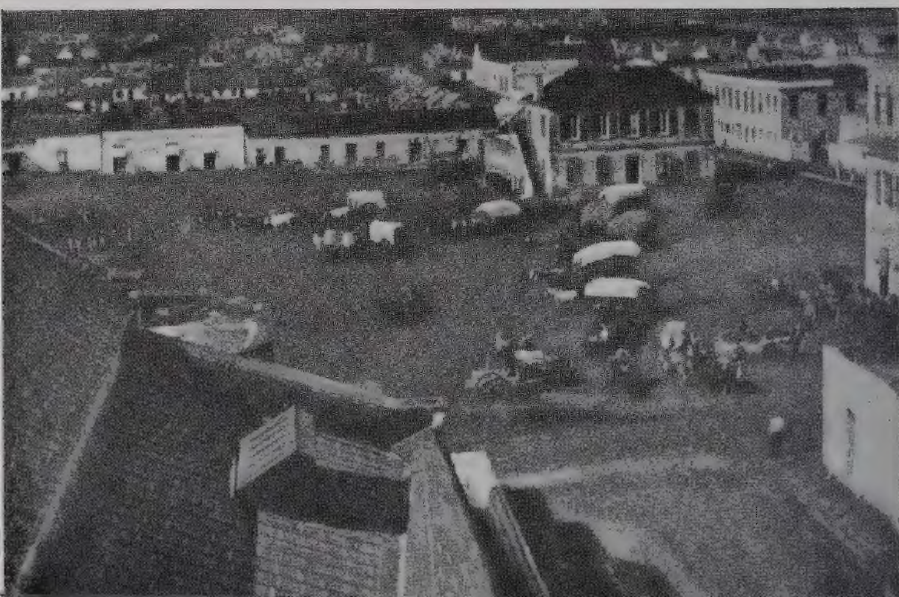
Looking west across Military Plaza from the roof of San Fernando Cathedral. Old Bat Cave is right center; low building to left is Governor's Palace. Hay wagons are on the plaza. Ted James Collection.
