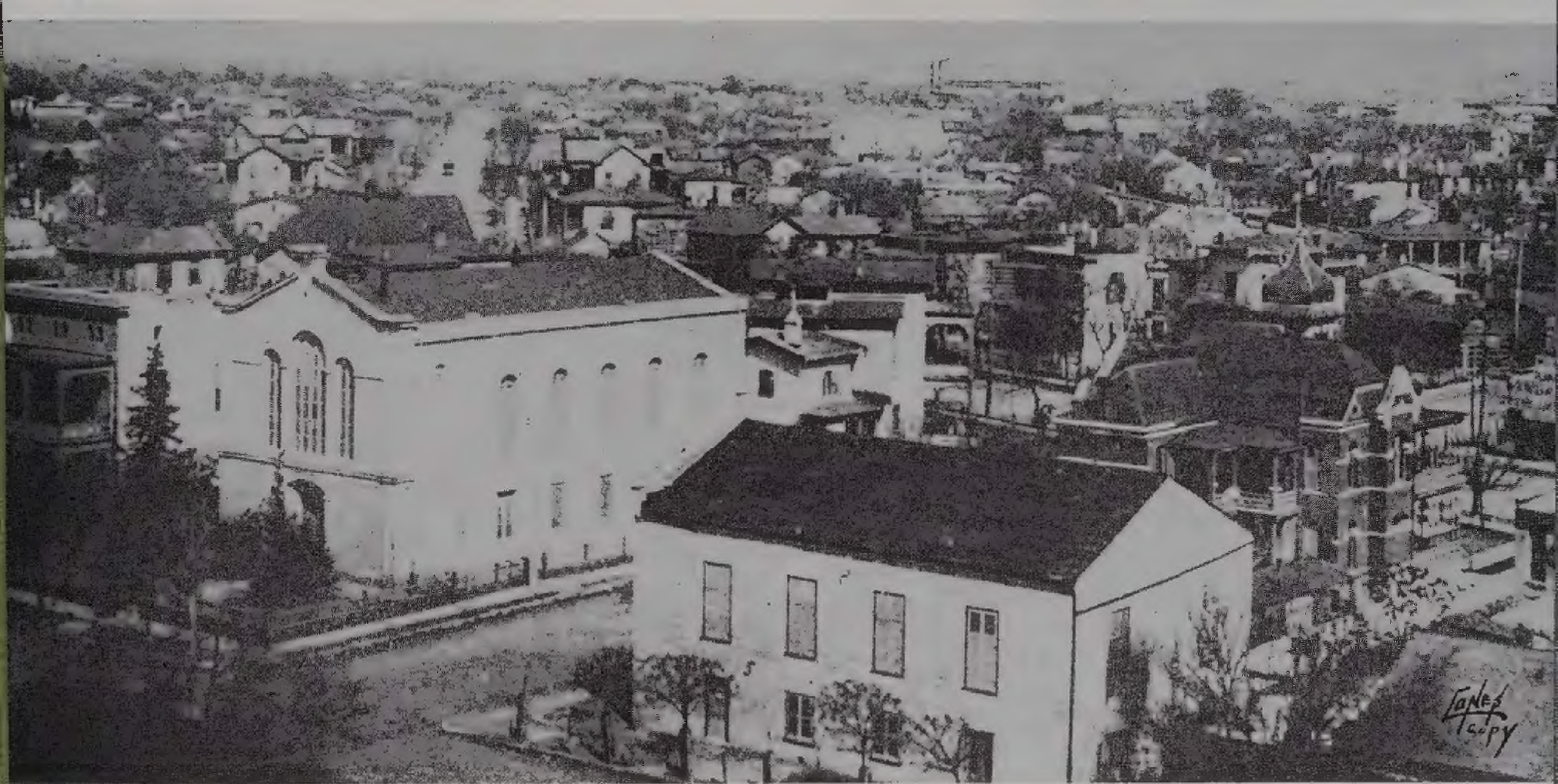
Looking northeast from the intersection of Travis and Jefferson streets. Buildings in foreground, left to right, old Michel home, now Porter Loring's, old Jewish Synagogue, Alamo Baptist Church. River Avenue, now Broadway, in distance. Albert Steves Collection.
