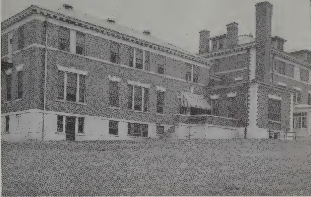
Now View of present Ossining Hospital from the South.
