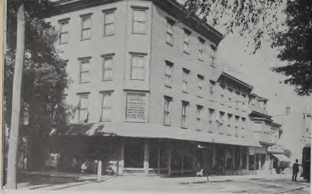
Then Corner of Spring Street and St. Paul's Place, N.W. Trees afforded shade and natural beauty.
