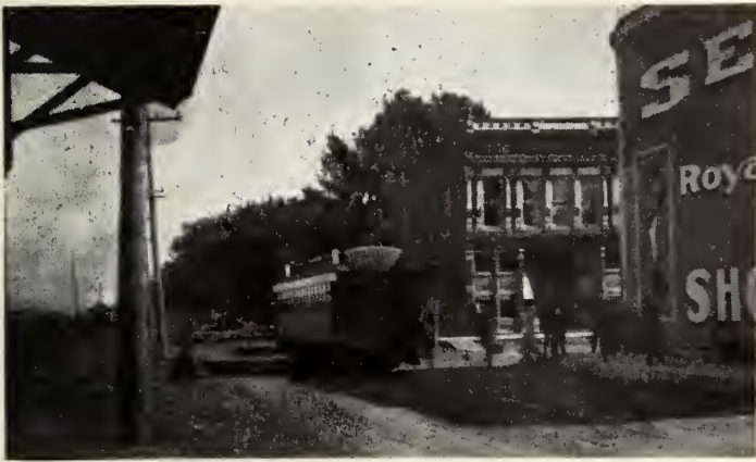
Above — Shroeder Boarding House
