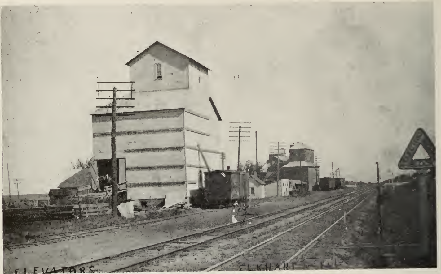
Elevators at Elkhart in 1907
