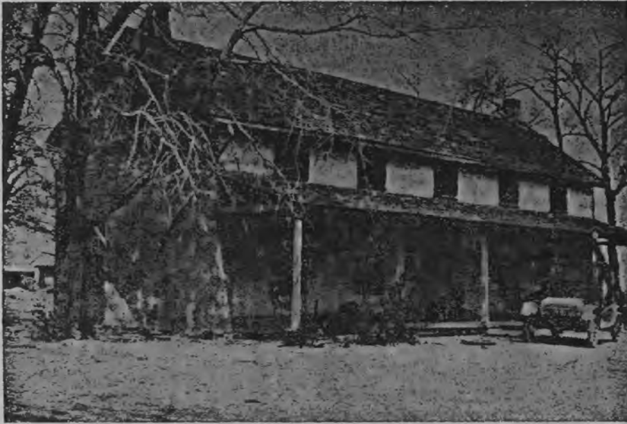
This is the front section of the Prowers house, as it stands today. Its walls are of adobe bricks that were made with grass and weeds as binder. The door and window frames were bought at Westport, Mo. ready cut.
