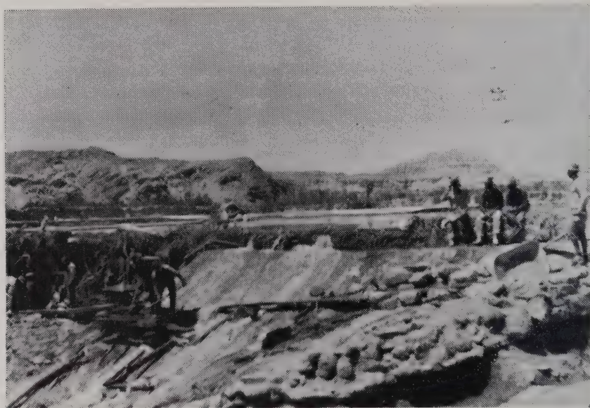
Dam in Fremont River, west of Bridge at Hanksville.
