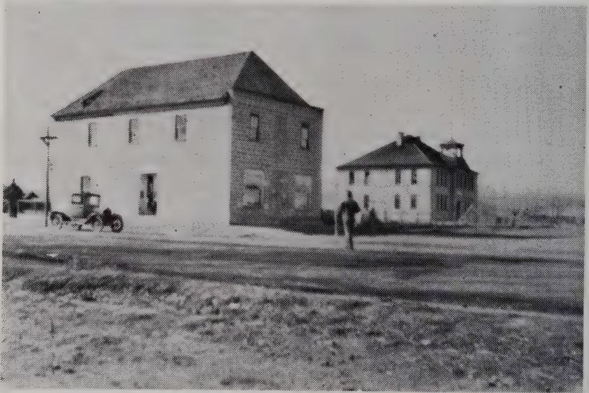
Old Court House Building and Old School Building
