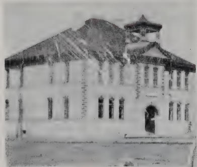
Loa Rock School House built in 1901-1902. Has been torn down and rock used for construction of new building.
