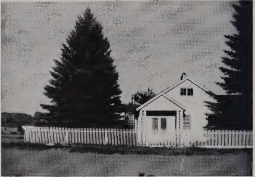
West View of U. S. Forest Ranger Station in Teasdale
