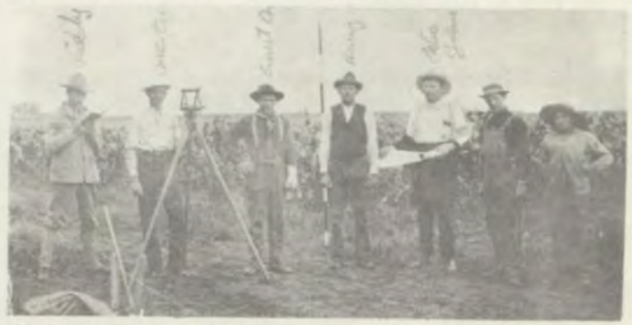
First surveying stake driven.
