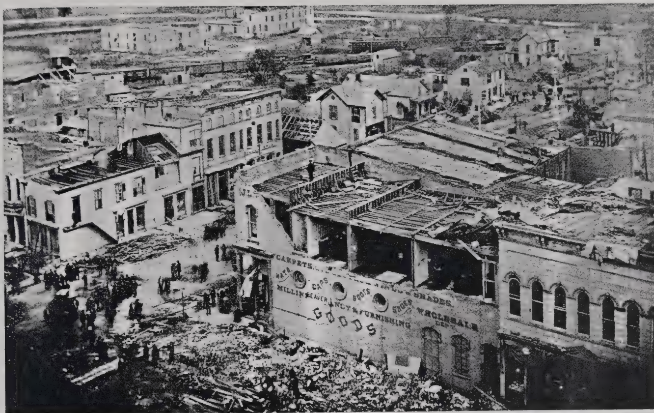
An outstanding picture of the havoc caused by the cyclone which struck Washington C. H. and Fayette County on September 8, 1885. The photographer was standing in the court-house tower facing the corner of Court and Main Streets.
