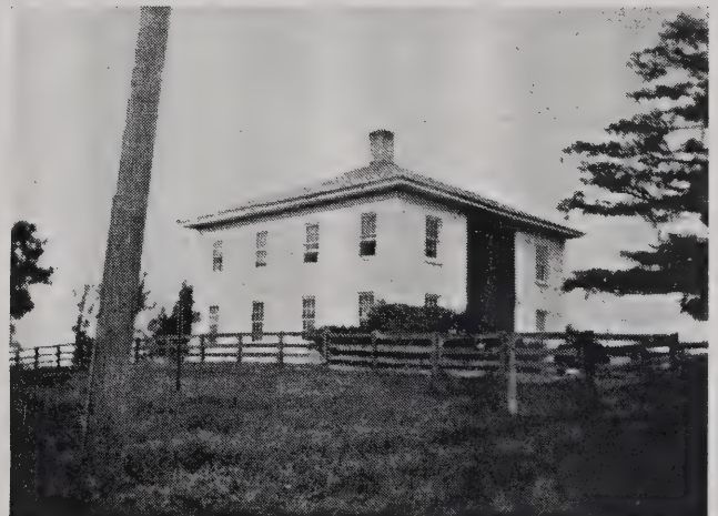
The chimney is in the exact center of this house and a circular stairway winds around it. Humphrey Hidy built it about 1846. It's on the Bookwalter Road.
