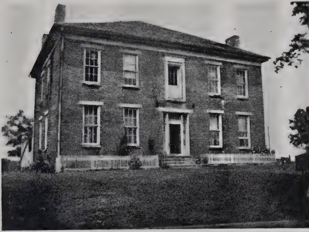
Built by David Persinger around 1840, this is believed to be the only house in the country with the old-type "balloon construction."
