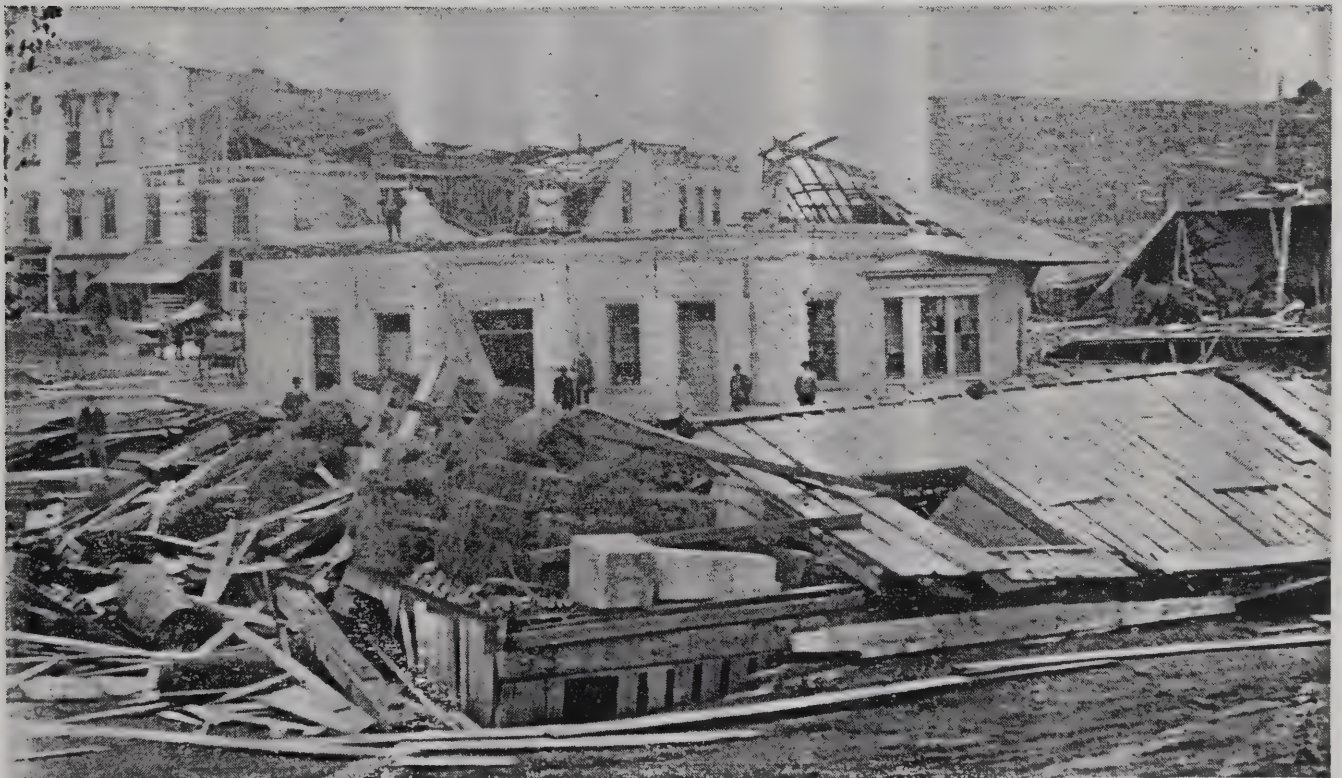
A picture of the C. & M. V. railway station showing the destruction in that corner of the city. The photo was taken with the camera facing the corner of East and Main Streets.
