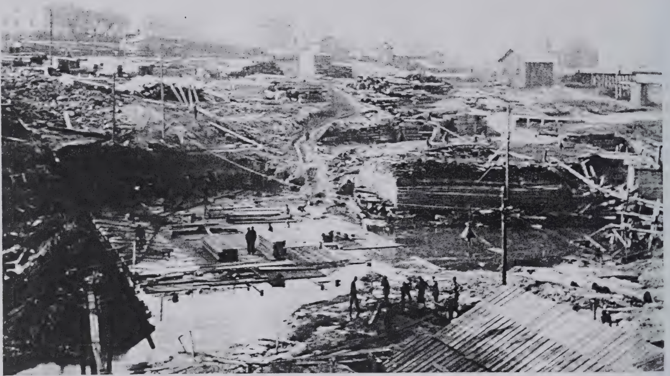
STARTING CONSTRUCTION OF NEWAYGO DAM
