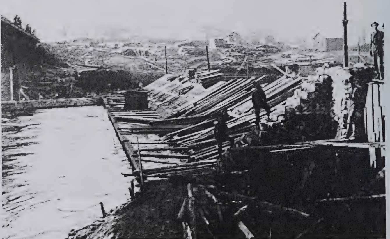
DAM PARTIALLY COMPLETED
