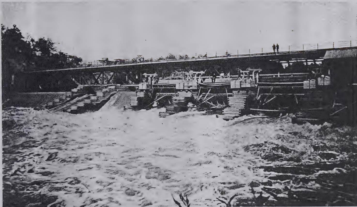
DAM COMPLETED AND IN OPERATION. Concrete facings were poured on Dam for added strength.
