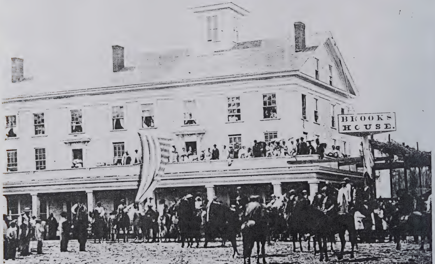
Brooks House - Burned in The Fire of 1882 Replaced by Courtright Hotel
