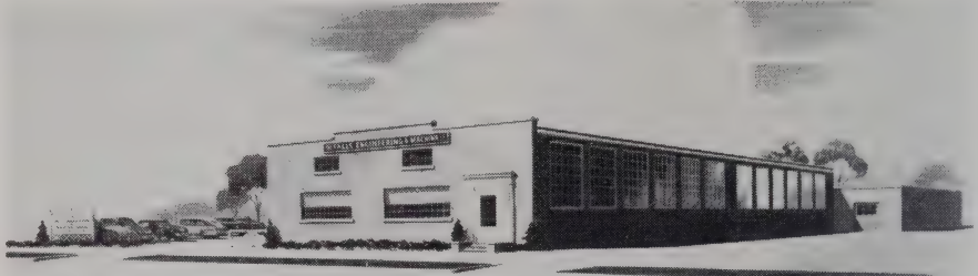
View of Falls Engineering Plant in Cuyahoga Falls
