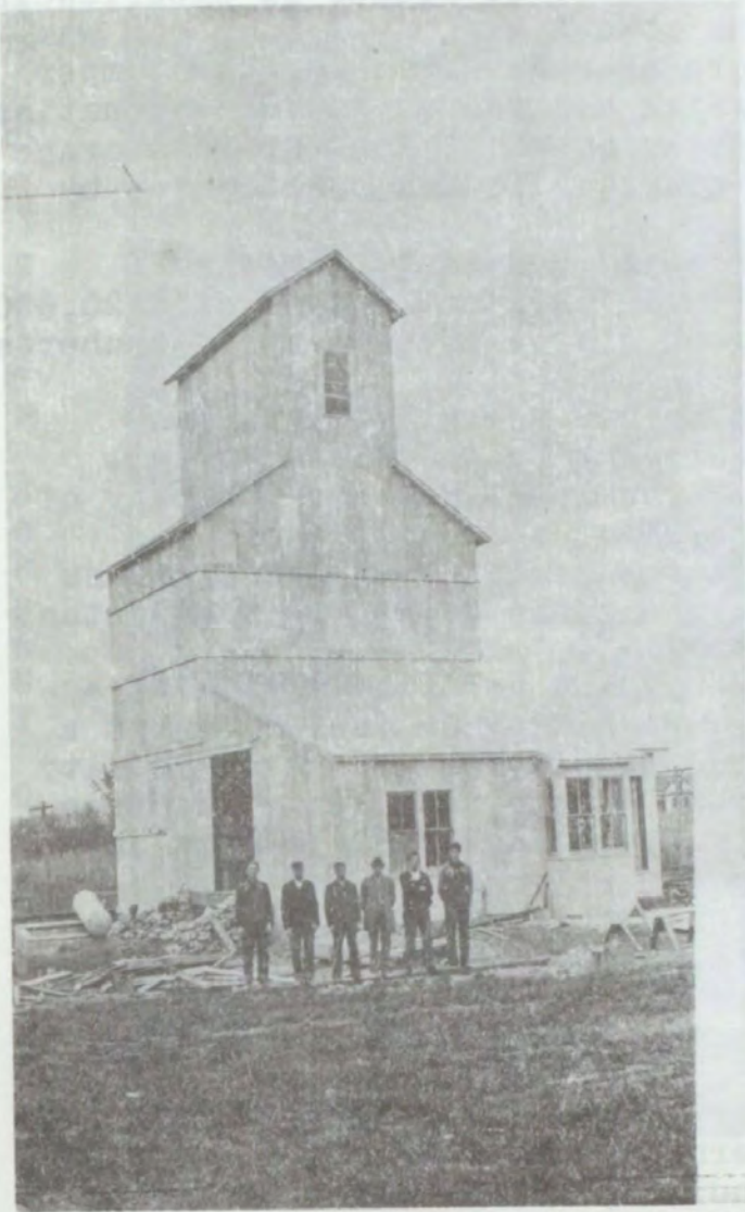
Original Archer elevator under construction.
