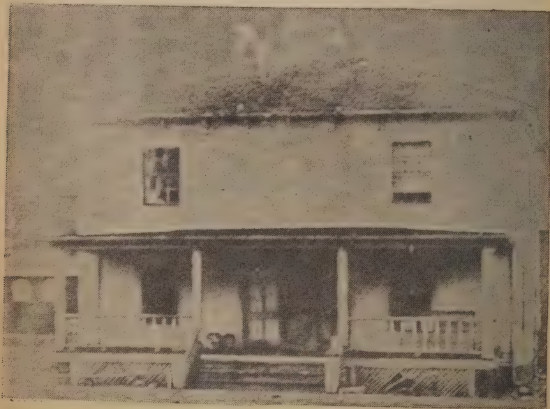
FIRST STATE HOSPITAL BUILDING, a farm house converted in 1864. Has been torn down. (Photo courtesy Osawatome State Hospital.)
