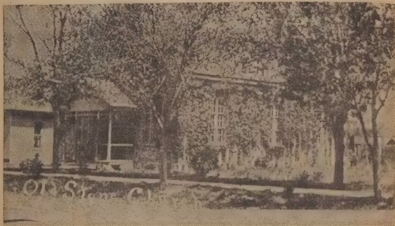
OLD STONE CHURCH, founded in 1859, and dedicated in 1861; erected by Rev. Samuel A. Adair. Being preserved by Osawatomie Historical Society. (From an old photo.)
