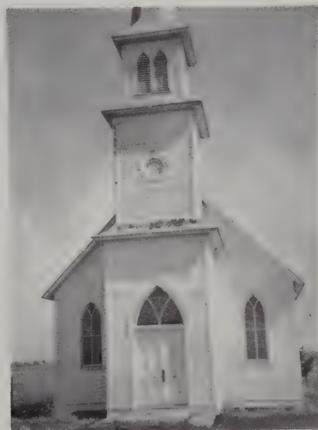
The small community Church once useful, now awaits the wrecking crew.
