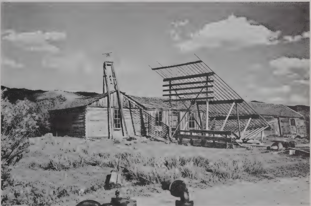
Old Bunk House and Office used by the Dole Brothers (Albany Land and Cattle Co.) at Buckeye Ranch. Note neatly dovetailed logs in bunk house and office.
