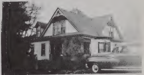
New House at Radichal (Plumbago) Ranch built in 1908.
