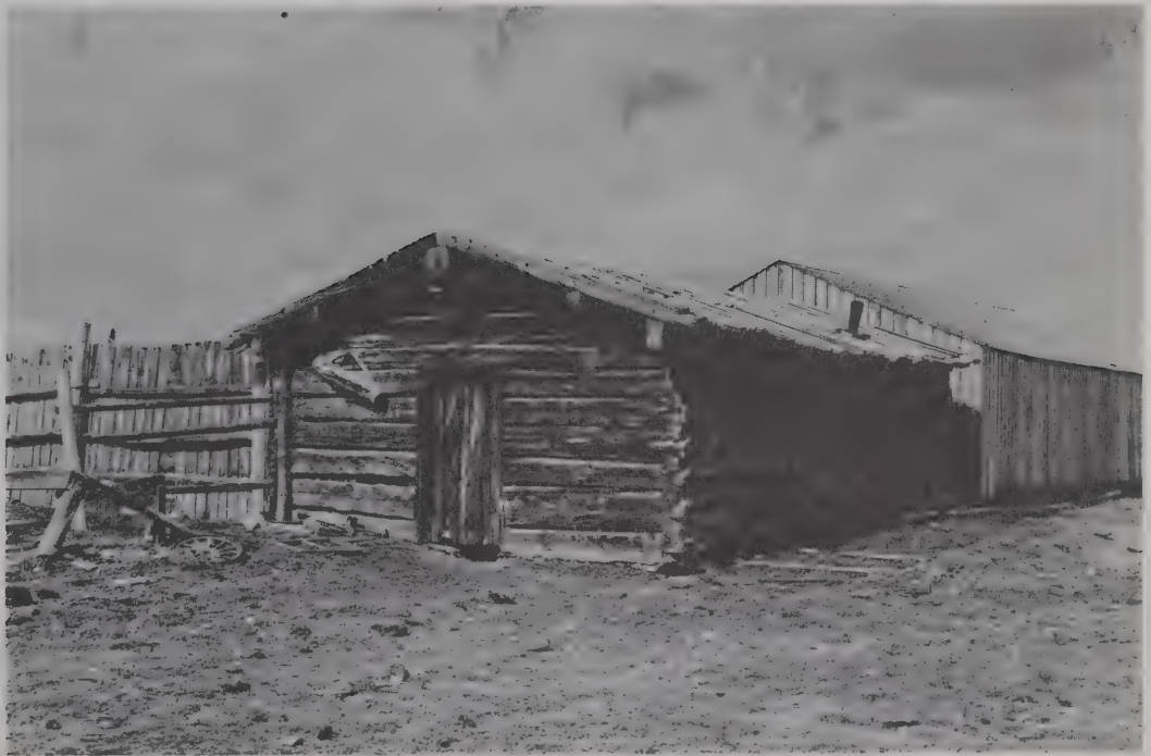
Mandel Blacksmith Shop. By courtesy Joe Kay.
