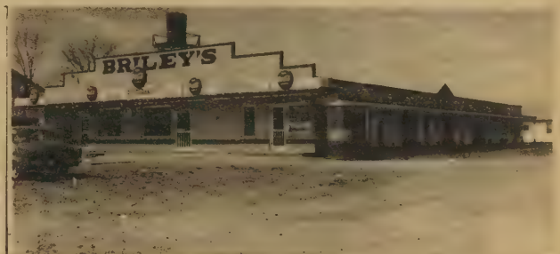
Photo above shows part of the addition of new Briley's Courts. Below the new modern restaurant, service station and courts.
