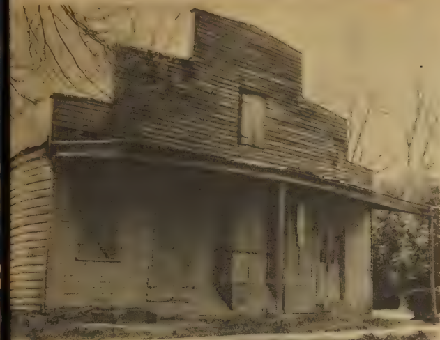
AN OLD-TIMEY STORE that is now abandoned, the Frank Brinkhaus store has a pair projecting showcases that displayed many wares in old days. Iron bars and hinges on battered doors and shutters are all hand wrought. The old Brinkhaus residence is next to the store, and is presently unoccupied. (Daily World Photo by Deville).
