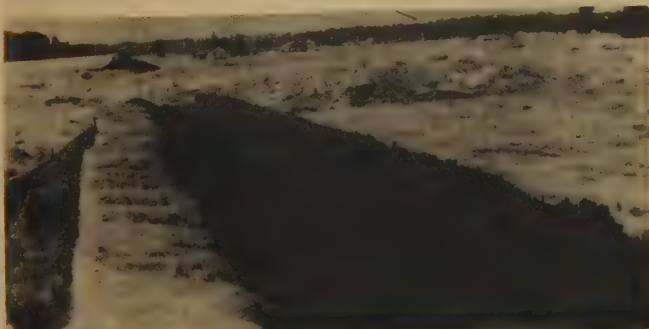
ANOTHER VIEW of 1927 levee crevasse at Melville, looking south as water pours inland. Row of sandbags on top levee in foreground was futile attempt to stave off disaster.
