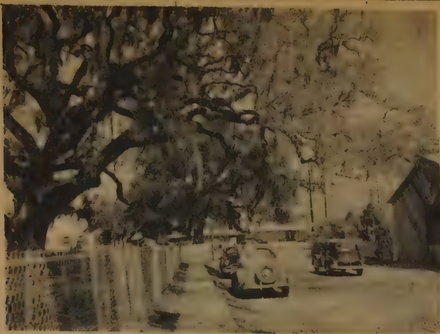
View in center of Arnaudville, looking towards the Bayou Têche bridge.
