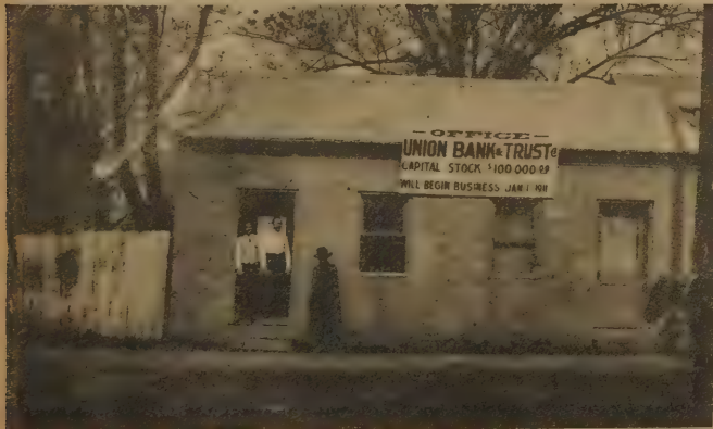
FIRST OFFICE of the Union Bank and Trust Co. was this small brick building on Bellevue Street, once the law office of Lucius J. Dupre and his son Laurent Dupre. A large placard on the building announces that the Bank will open for business Jan. 1, 1911. Standing on the steps are Jean Jacques Perrodin (called "Jack") who was first cashier of the bank, and James Vidrine, his assistant. This building was used for a year during construction of the Union Bank Bldg. at Bellevue and Court sts., presently the home of the Planters Trust and Savings Bank, which will move this year into a new building now being constructed across Bellevue street from the present structure.
