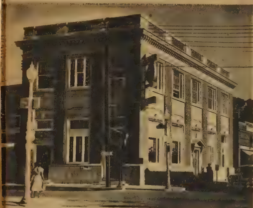
Old Building — Erected 1905.
