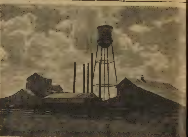
SUGAR FACTORY on Augusta plantation at Barbrech, silent since 1946, stands today as a relic of Old South. The plantation dates to Spanish grants. It was formerly a part of St. Peter's plantation. Augusta plantation was owned and operated by August Hamilton de Lesseps from about 1900 to 1905. Plantation got its name from his wife, who was August's daughter. Upon August's death the plantation was operated by an investment company, his son, Hamilton deLesseps, as president. Hamilton converted old syrup mill into a refinery and continued operations until 1910, August then went into hands of the Haas Investment Co., with Dr. W. D. Haas of Bunkle at the head. The Augusta sugar factory ceased operations in 1946. Sam Haas is now president of the Haas Investment Co., owners of Augusta. Other members are W. D. Haas, Jr., Mrs. Roy Harrison and Franklin Mikel.
