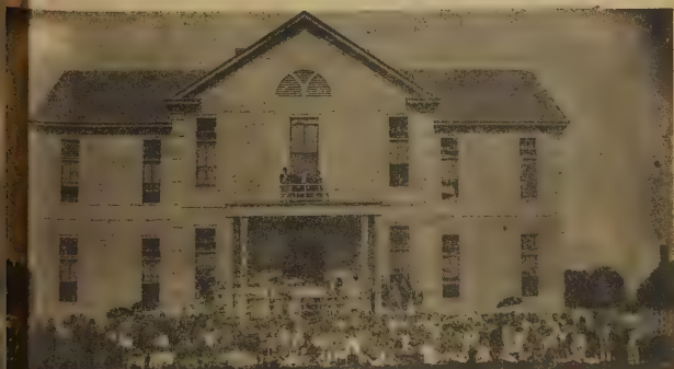
LANDRY HIGH SCHOOL , photographed May 11, 1900. At the time, it was located on West st. at the site of the present St. Landry Clinic. The building was later moved to Academy st. and became the Opelousas Negro High school. It was abandoned years ago when the present J. S. Clark school was built, except for adult education classes and various gatherings. Photograph was originally the property of Ludie Prados, and is now owned by Mrs. James Prados.
