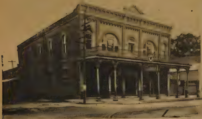
BORDELON'S GARAGE taken shortly after remodeling from a grocery store, in 1916. Note the iron balcony rail on top of the gallery.
