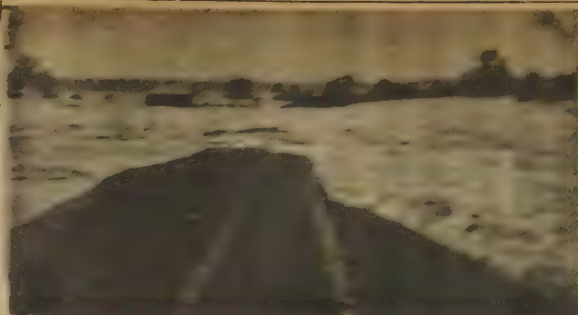
ODENBURG CREVASSE, taken at 9:30 a.m. May 12, 1912. This is considerably north of Melville, but Atchafalaya water flowed down, flooded the town well before the levee broke near here. Somebody pencilled the following notations on the back of this picture. "Wed., May 15, 1912, water started to come in yard. Thurs., June 20, water left yard. Moved to depot May 20, 1912. Moved back home June 11, 1912. This taken May 19, 1912, at 9:30 o'clock, lacked eight inches of being in house."
