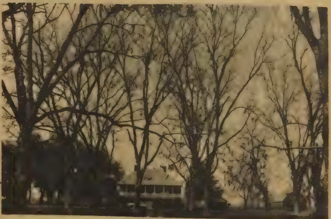
Near Opelousas, off the road to Ville Platte, is one of the loveliest plantation homes in the section - the old Powers place, now owned by Harvey Phillips. Built in the typical "River Plantation" style, with lower floor of brick and weather-boarded upper floor, fronted by a double gallery, the home is built in a grove of magnificent live oaks, from which the name of plantation was derived. A long avenue of oaks leads to the house adding to the setting. Brick pillars on the lower floor support the upper gallery, with its slender cypress columns. There are several homes in the immediate vicinity of Opelousas of this same type of construction. The original batted shutters with their hand-wrought iron hardware add to the general beauty of this old home. The house was at one time occupied, and had fallen into a state of considerable disrepair, but has since been gradually repaired by the present owners, who are restoring it to its original condition.
