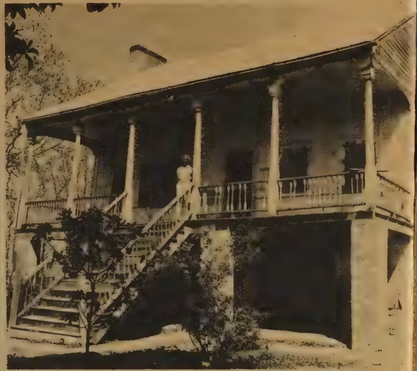
PLANTATION HOME of Jack Compton, once a prominent planter of St. Landry Parish, is situated in the East Bellevue section of St. Landry, near Opelousas, on the Opelousas road. It is now owned by Isaac Lewis who is pictured standing on the gallery. The lower floor of brick supports the upper living quarters, as is typical of this period. Once a lovely home, it has finely panelled sections on the gallery, woodwork and nicely turned railings on the central staircase of the exterior. Slender cypress pillars support the upper gallery; the lower pilasters are squared brick. It is situated on a slight rise, and once had an avenue of oaks in front of it, traces of which are still standing. (Daily World Photo by Deville).
