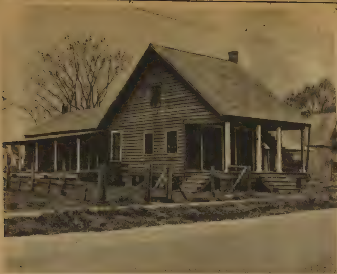
PAINTED BARN RED , it has for many years been to this writer one of the most attractive homes in Grand Coteau, with French doors opening on the front porch, from which extend a flight of open stairs that ascend to the attic. Known as the "Acadian House", this style of building is fast fading from the picture, and one seldom sees a home in as good condition as the house pictured. It is owned by Mrs. Chattrillon, who lives in a larger home around the corner.
