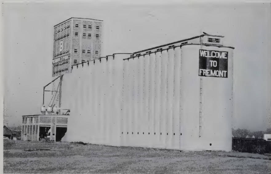
West Central Co-Op Elevator, 1956
