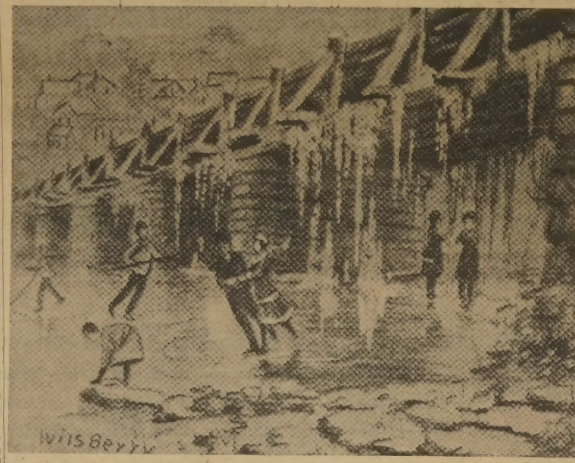
EEL RIVER AQUEDUCT —The foundations for this strange structure remain in the bed of Eel river back of the old brewery, where a hundred years ago the Wabash & Erie canal crossed the river. This picture is from a painting of it by Wils Berry, a local artist of some years ago. Canal boats were towed across the river at this point to continue angling across the westside to Water street, whence the canal went west, crossing the Wabash river at Lockport. Mr. Berry's painting shows skaters on the river below the aqueduct, which has dripped water that froze into icicles.
