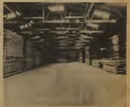
An interior view of the main storage shed. Here the hardwood is arranged as to quality and type of wood, making for efficiency in filling orders to dealers.
