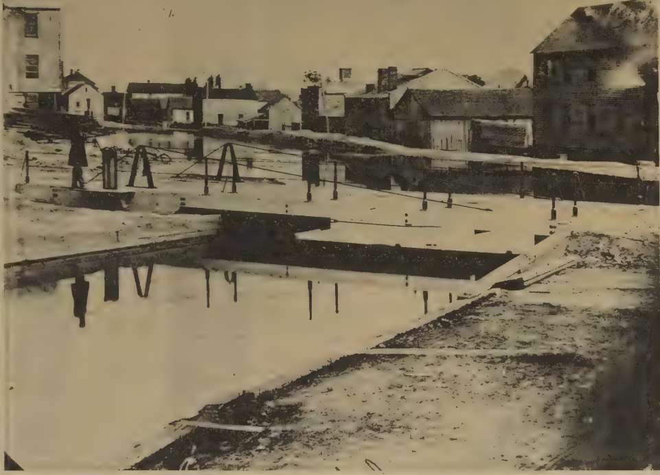
FIFTH AND MARKET—This 1858 picture taken at Fifth and Market streets shows the canal in its last days. The draw bridge paralleled Market street. The building which housed the Henderson furniture factory is at the right edge of the picture. The wide spot in the canal beyond the bridge is the old turning basin. The present Labor Temple building is in the point beyond the man standing at the crank which operated the bridge. The canal trails off to the right background up what is now Erie Avenue. Workmen digging at Fifth and Erie still run into planks which were part of the installation seen in this view, which reveals the construction that followed the canal banks through much of the city. The canal, of course, turned at Fifth and went north to cross Eel river back of the brewery property on the aqueduct.
