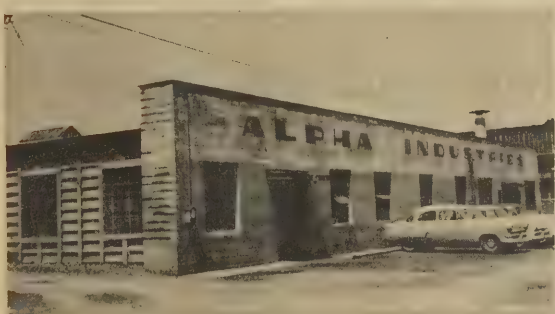
Still at its original site, Alpha Industries has grown from a plant of 8,000 square feet to a firm whose ground and buildings cover 6 acres, many of which were acquired from the old Boyer plant.
