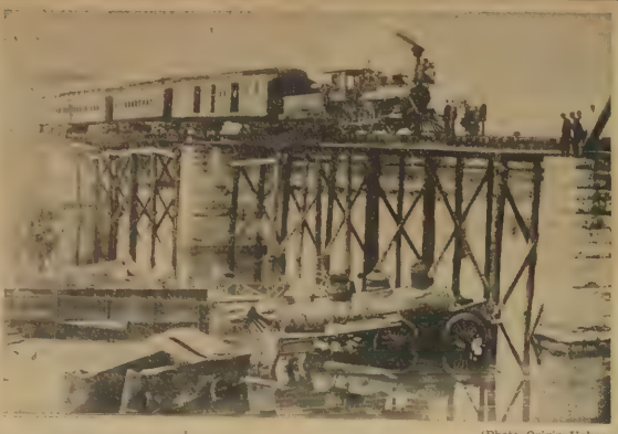
LC BRIDGE WRECK—The engine and fireman of this train met death in this 1882 railroad accident. The engine and following five cars went into the Wabash river when the bridge gave way beneath it. The debris of the wrecked train remained in the river bed after the bridge was repaired and returned to use. Two spans of the bridge, twice since completely replaced, went down. (Photo Origin Unknown)
