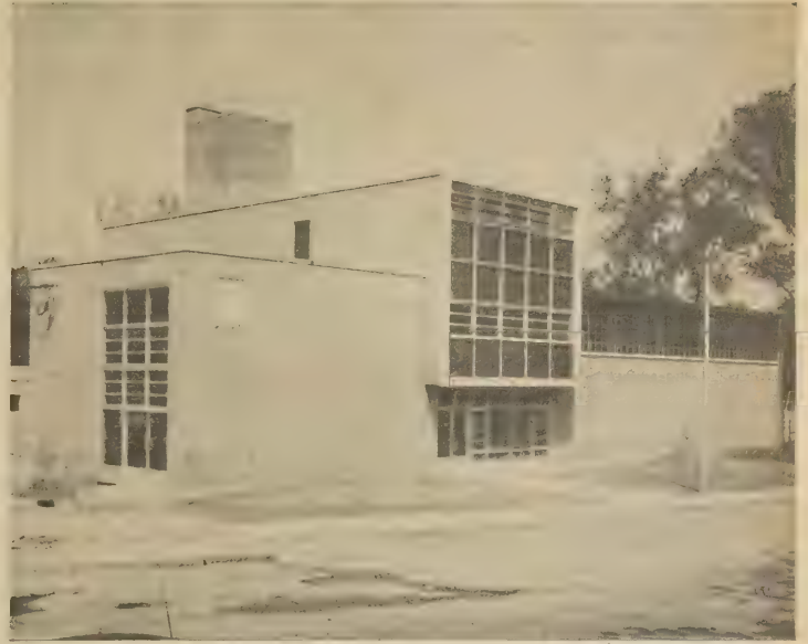
NEW LOGANSPORT WATER PLANT
