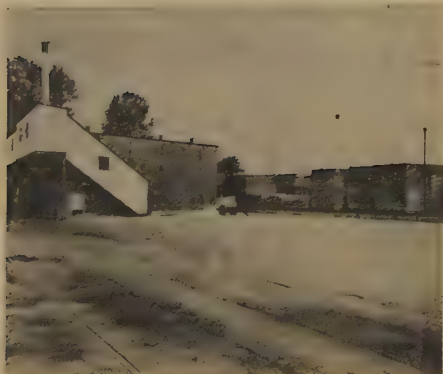
The dry kiln where the lumber stays from two days to two months, depending upon the species, thickness and degree of dryness.
