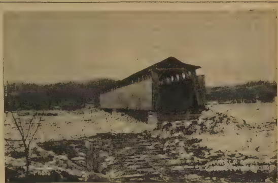
LAST GEORGETOWN BRIDGE—The heavy ice movement from Eel and Wabash rivers stacked up against the old covered bridge at Georgetown in 1912, with this result. The rest of it later removed and the present bridge constructed. Pieces of the smashed span can be seen mixed up with the ice in the foreground.
