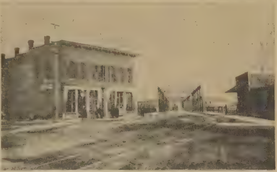
OLD MARKET ST. BRIDGE—It hasn't been so long ago that this sight was familiar to westside people going east across Market street bridge. The Frank Kienly saloon for years operated in the building on the left, a barber shop on the right. Both these structures were removed before the new concrete bridge was put in during 1930. The street car track is shown following the south side of the bridge roadway. It was not necessary in 1930 in the rebuilding. (Courtesy Mrs. Walter Foskett)
