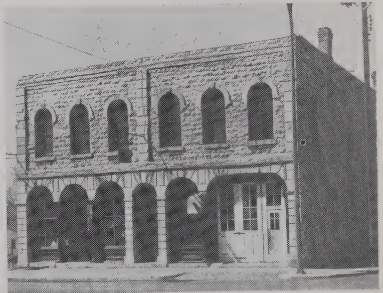
The gray stone Williams building at the southwest corner of Second and Commercial streets was built by the late T. E. Williams following the great Hudson fire of 1866.
