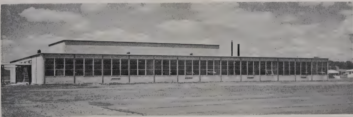
New Edward P. Rock Grade School Building in Quality Park Addition, constructed 1956-57.
