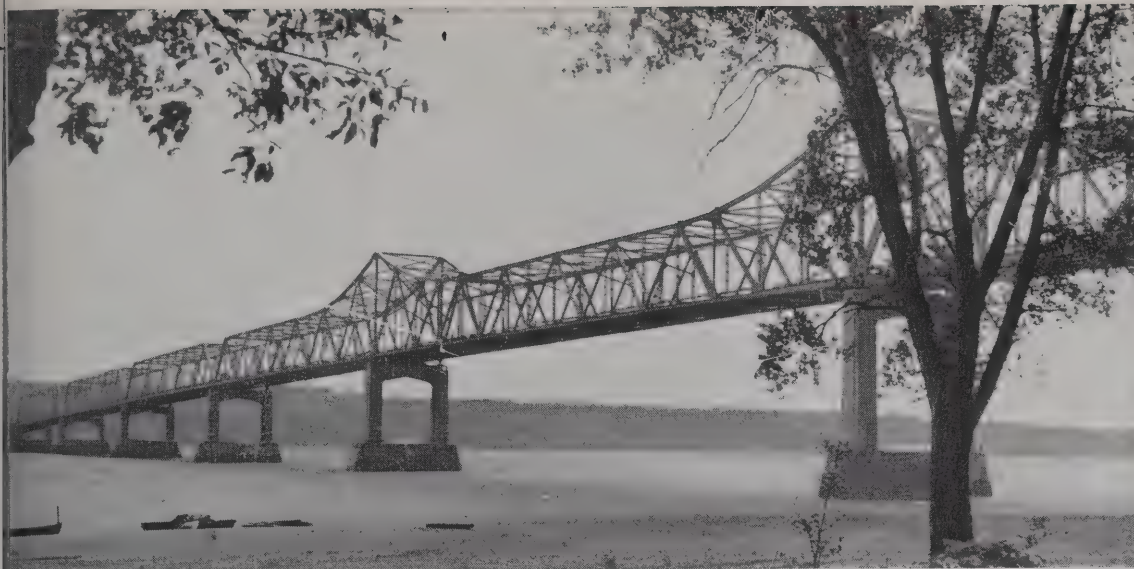
The new Minnesota-Wisconsin Interstate Bridge opened in November 1951.
