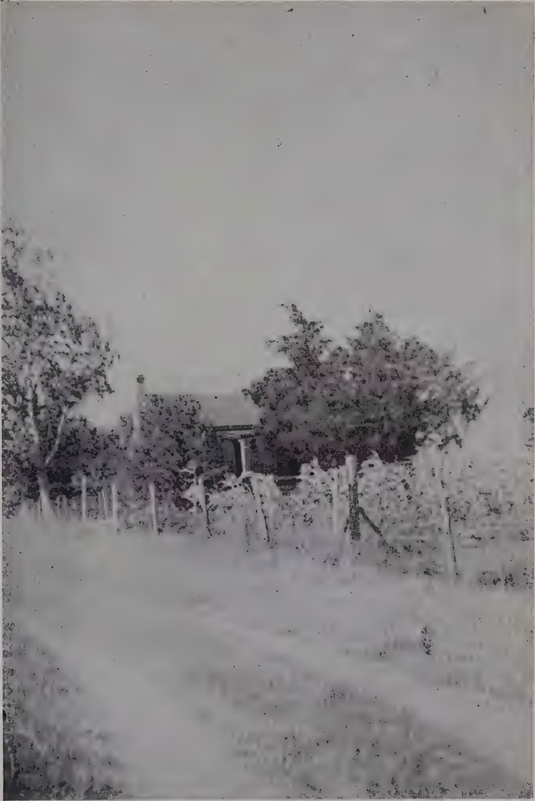
This famous old home was built by the father of T. G. Sampson at an early day. It is said to have been built without nails, wooden pegs being used. The bricks were made by slaves on the place, the lumber brought in by ox-cart. Old-timers say this house had portholes, for protection against the Indians. The elder Mr. Sampson carried his bride across this threshold. Tom Sampson was born here.
