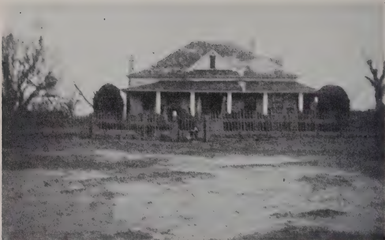
Home of Miss Ethel McKinney, Jones Prairie. Built on site of original home. One of Milam County's most representative families.
