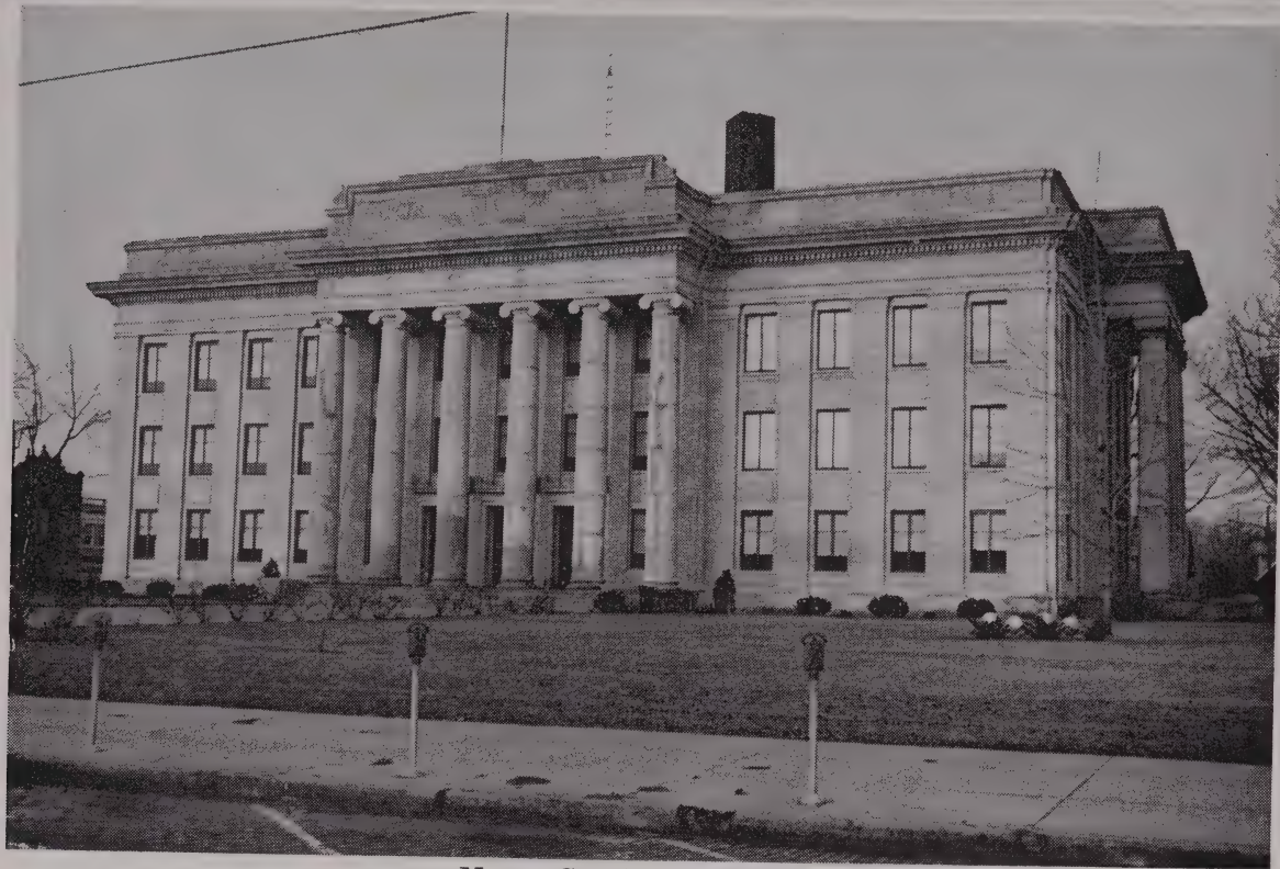
Mercer County Court House
