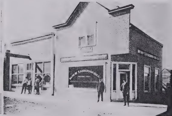
The old bank of T. Anderson-Oie and Co., which became the Citizens State Bank in the early 20's.
