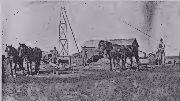
One of the first tasks confronting the homesteader was the digging of a well. This 1916 photo of a high derrick, taken by a traveling photographer, shows one of the methods used. Ben Larson, an unidentified man, and George Skerritt are on the scene.
