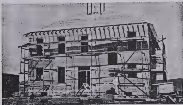
Whitetail school under construction in 1915. This school is still in use.
