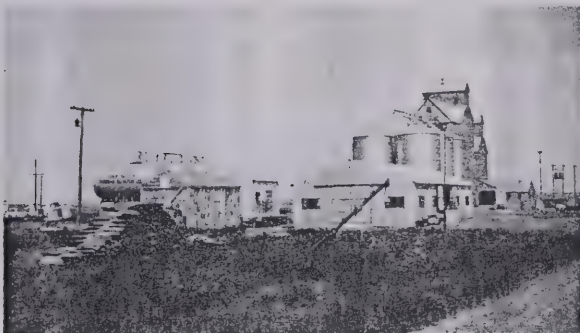
The Farmers Elevator and storage tanks in Four Buttes.
