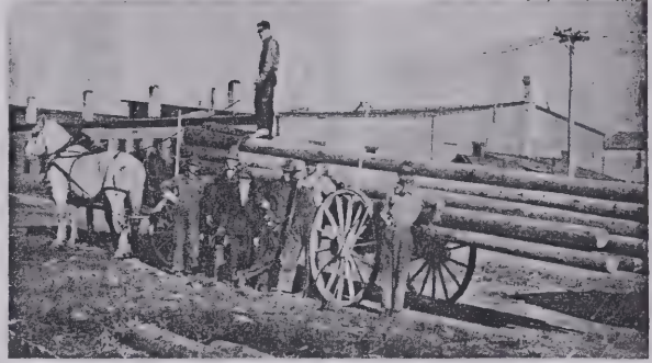
When Gutherie Construction started west with the steel, telegraph poles were also set. This picture, taken in 1914, shows F. A. Sunderhauf, driver and owner of team, and from left to right, unknown, Carl Renner, Fred Bates, Ed Bulondie, (line man), unknown, Jack Harvey (line man).
