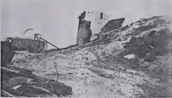
This is all that remained of one of the two Four Buttes elevators after the fire of 1944. Note the pile of wheat and rubble.
