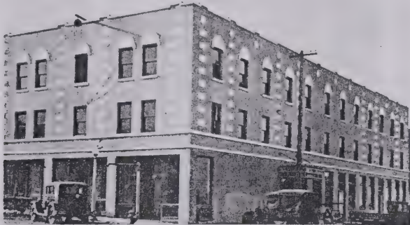
Gorham Hotel, constructed in 1928, standing on the site previously occupied by the city hall, fire hall, and jail.
