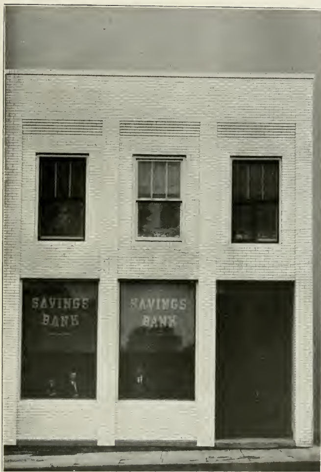
BRIDGEWATER SAVINGS BANK
