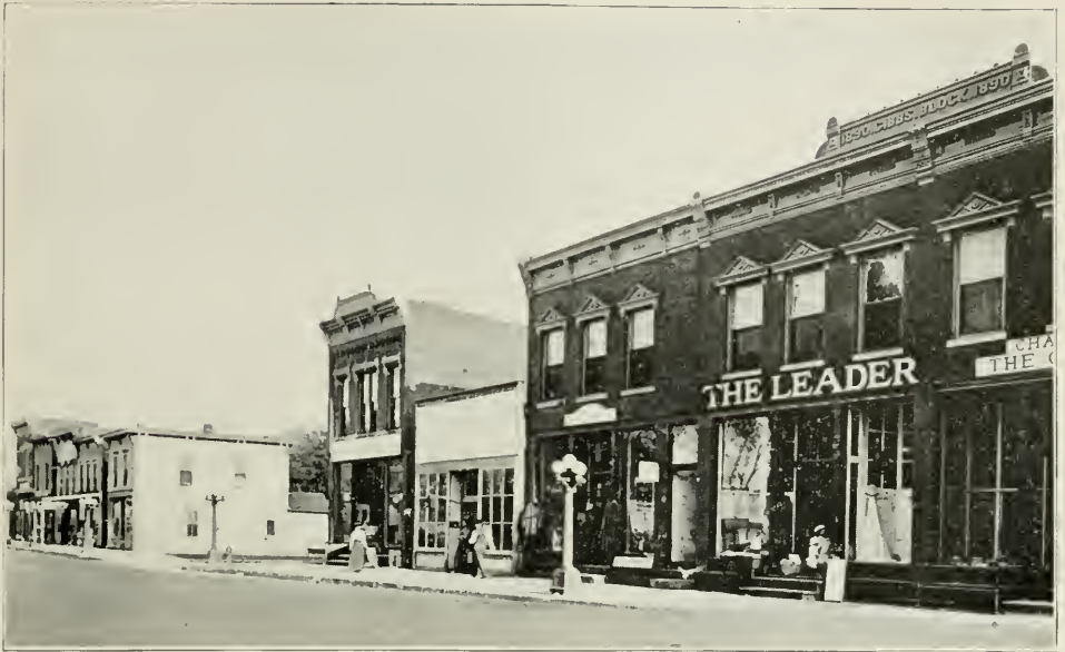
SOUTH SIDE SQUARE, GREENFIELD
