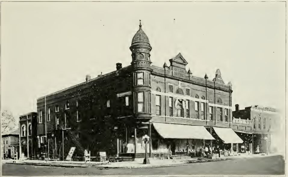
OPERA HOUSE, GREENFIELD
